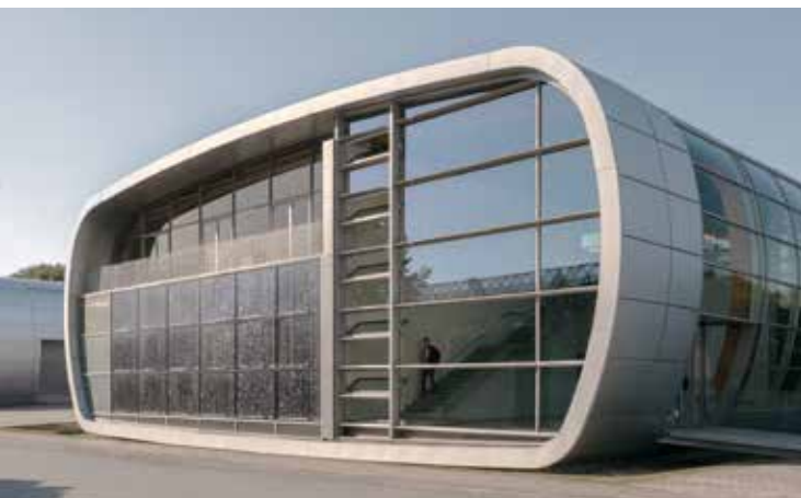
GRAU, Office and industrial building, Rellingen, Germany (1998)
